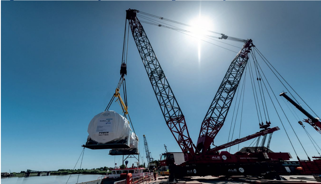
Figure 3.4: The Keadby 2 CCGT arriving via Keadby Wharf in 2020
